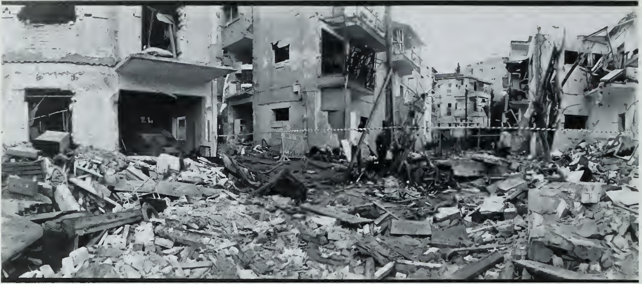
Fig. 4-7. Photo of damage caused by a Scud strike.
